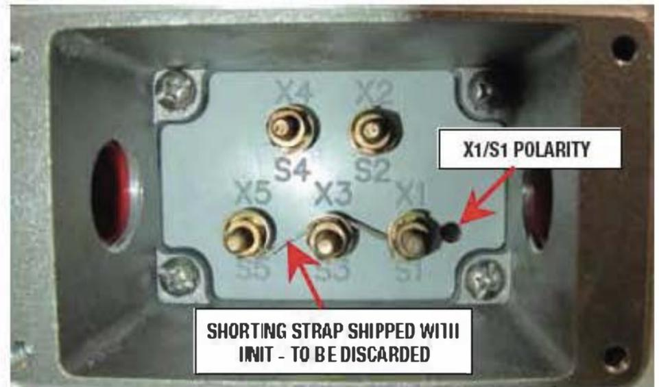
When wiring a multi-ratio SBCT, only connect to the desired tap and leave all other unused taps alone – do not short any unused tap.
